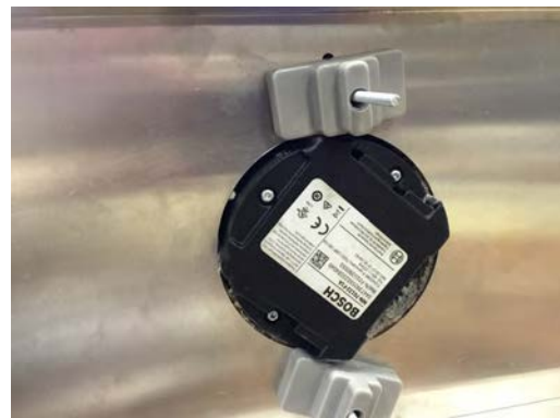
Example installation: FLEXIDOME camera clamped to MNT-ICP-FDC, with MNT-RIS-FDC, on top of ceiling tile
