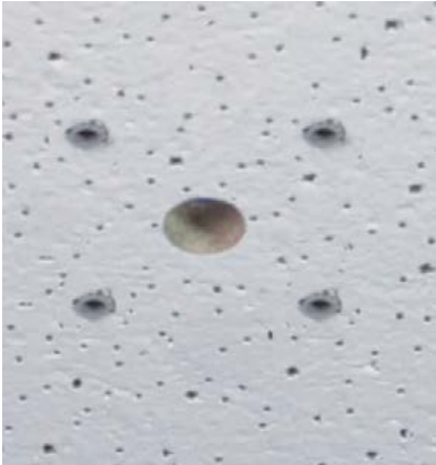
Fig. 14: Holes ready for mounting
