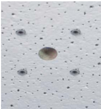
Fig. 16: Holes ready for mounting
