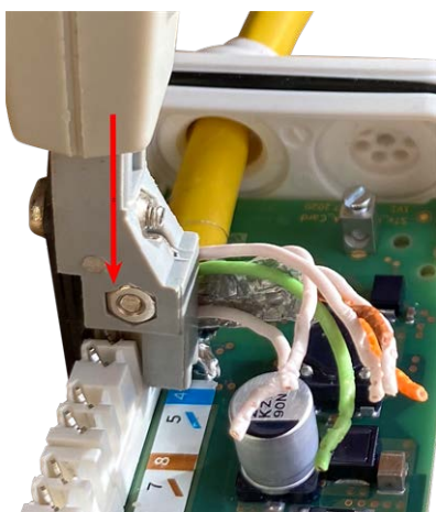
Fig. 26: Network wires connected using LSA+/Krone tool
