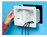
1 Cut Top hole in wall for the TV. Cut Lower hole directly below the top hole, close to an existing outlet.
