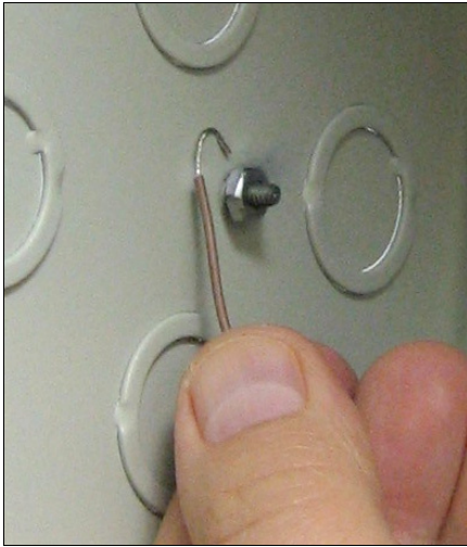
Fig. 5: Connect ground wire to grounding screw.
