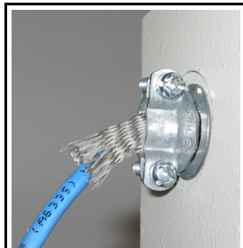
Fig. 6: PANEL EXTERIOR: Both the Ethernet cable and the braided shield must be grounded to the panel enclosure by the cable clamp.
