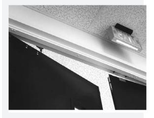
The 600 Coordinator and Filler are mounted on the soffit and painted to match the frame. The maximum projection of the hold open lever and trigger is only 1-1/8", thus the Coordinator and Filler are virtually invisible and appear to be an integral part of the frame opening.
