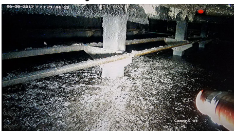
In-Use Robotic Sandblasting
