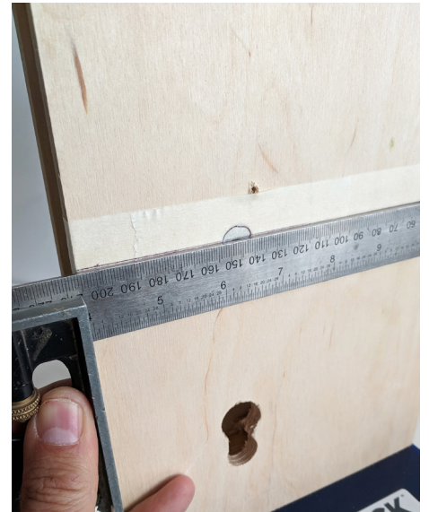
5. Apply masking tape to the door and draw a horizontal and vertical line through the centre of the spindle hole.
