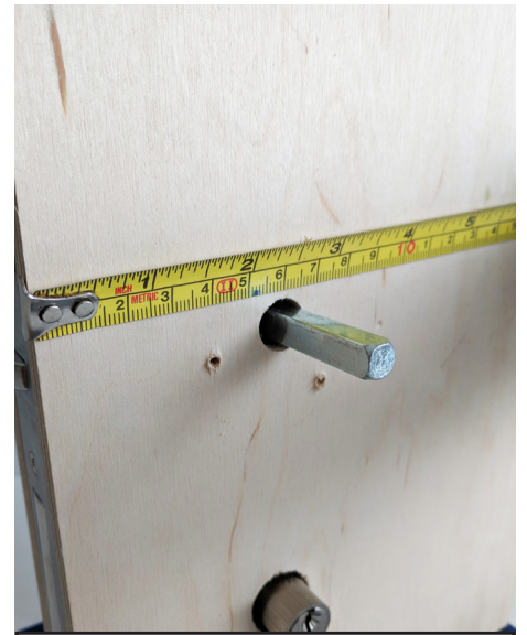
2. Check that the backset distance is at least 50mm, in this instance it is 60mm. If in doubt, tape the template to the door and make sure the lock will clear the door stops.
