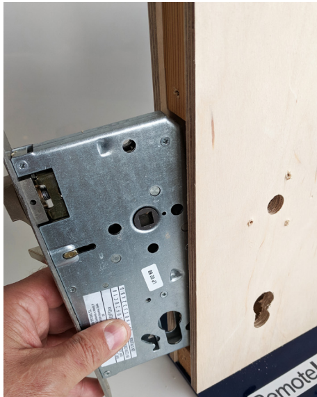
3. Remove the spindle, keyed cylinder and mortice from the door.
