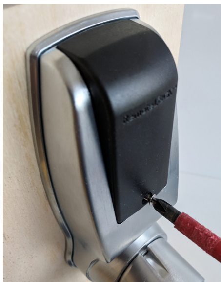
14. Finally, fix the plastic cover on using the screw.
