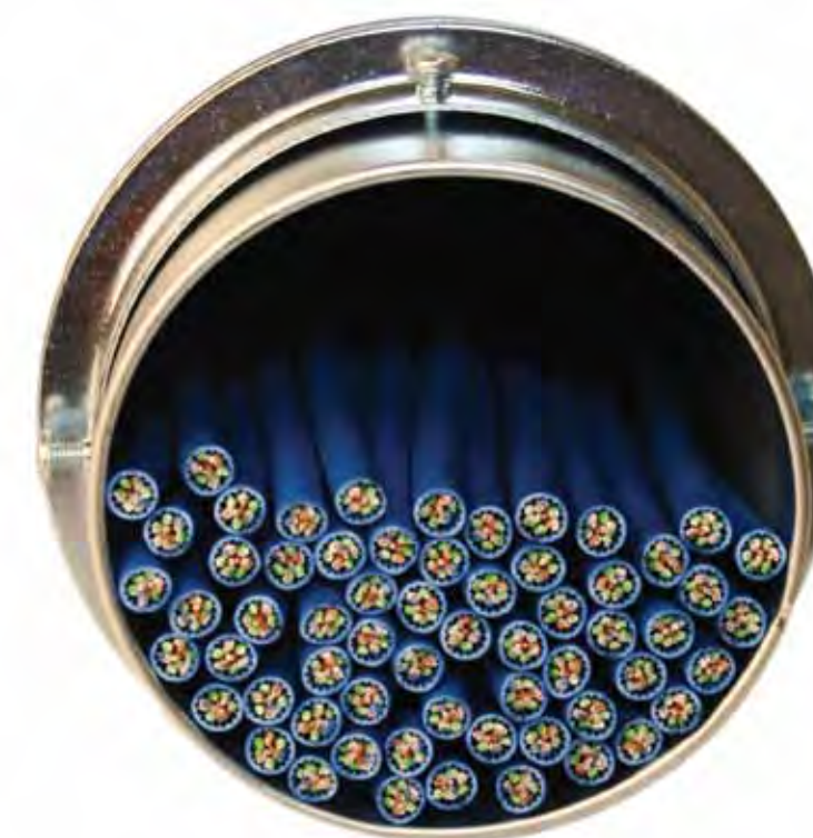
Typical 0.325" CAT 6A cable allows 61 cables in 4" conduit at a 40% fill rate.
